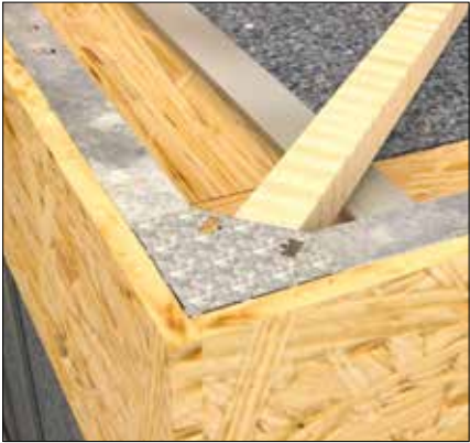
After laying out each firring start with the hip positions. Place firring into the joist hanger corner and align with the 2 tabs on the corner profile
