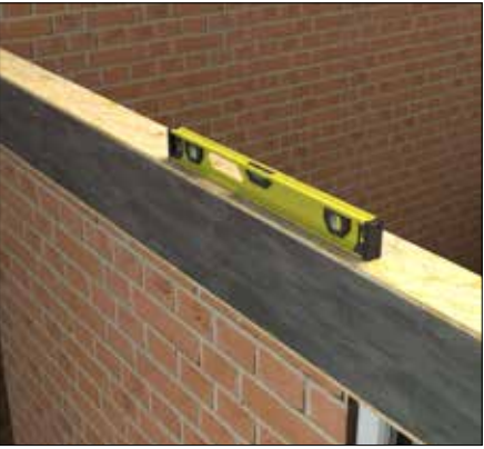
Once square, ensure the beam is level in both width and projection before fixing.
