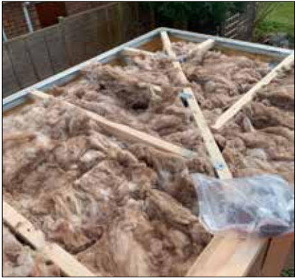
Before fitting the OSB decking fill the gaps between the firrings with insulation.
