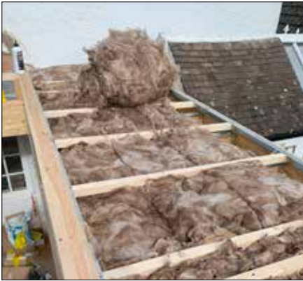
Before fitting the OSB decking fill the gaps between the firrings with insulation.
