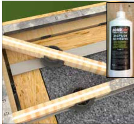
Before placing OSB deck, use the glue provided to place a line on the timber firrings that the deck will sit on. Also glue any joints in the OSB as you proceed around the roof.
