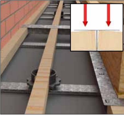
A t-shaped ridge plate may be included in your job. Place it in position and fix down through the ridge plate into the batten using 2x NPS050 on each batten.
